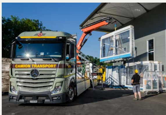
Collection by boom truck
